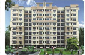
PRINCE RESIDENZIA, SRIPERUMBUDUR (440 Residential Flats), 5.81 lakh sq.ft.
